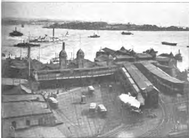
FOOT OF WHITEHALL STREET AND GOVERNOR'S ISLAND, FROM ARMY BUILDING.
